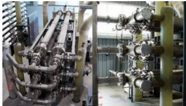
Fig 10 – DWEER rack on a 15 MLD line (Calder pictures)
